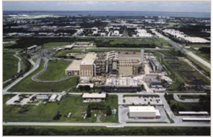
The waste-to-energy plant in Pinellas County, Fla., processes up to 3,150 tons of solid waste daily and generates 75 megawatts of electricity per hour—providing enough power for the plant and approximately 45,000 customers.
